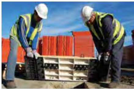
Road Plate: 59" L x 19.7" W / Weight - 96.8 lbs. End Section: 59" L x 19.7" W / Weight - 50.6 lbs.
